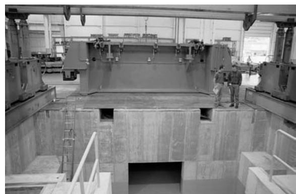
Press bed ready to be installed onto foundation piers.
