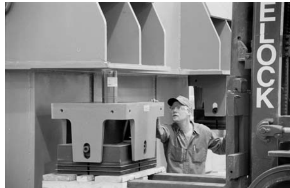
Isolators being lifted into place.
