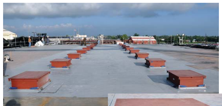
Installed isolator and arrangement on deck
