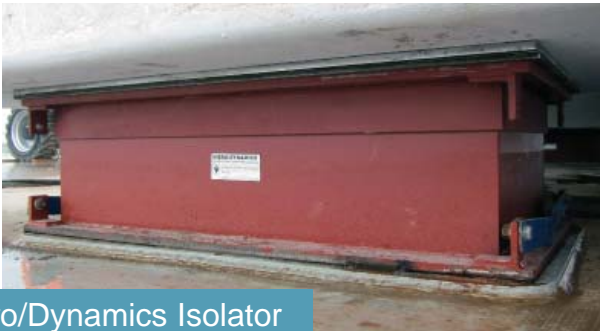
Concrete Plinth supported by the Isolators
