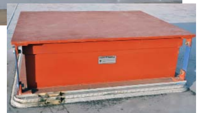
Installed isolator and arrangement on deck
