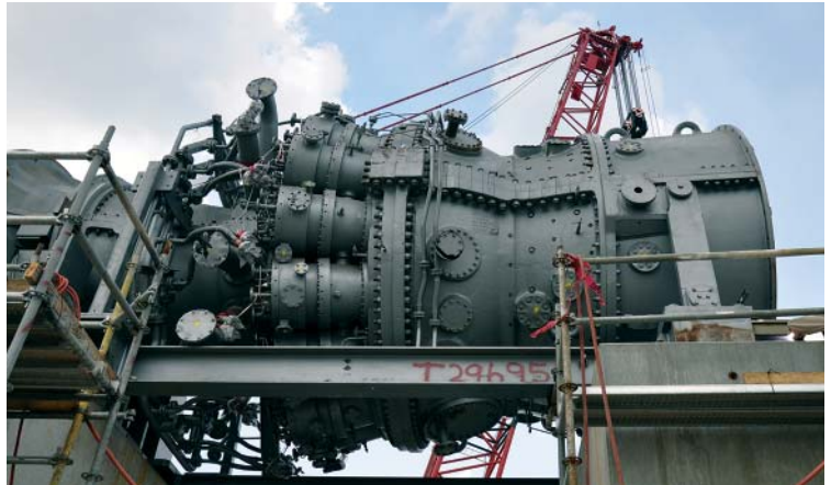
Assembly of Turbine on the top of the Plinth
