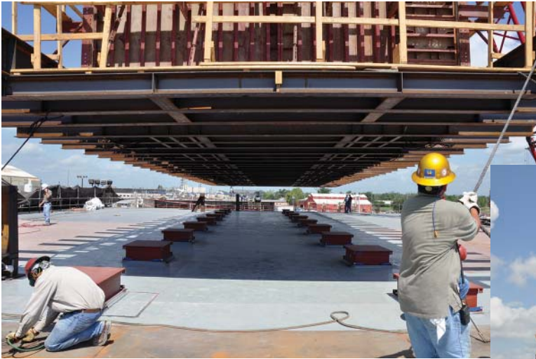
Plinth form-work being lowered onto the Vibro/Dynamics Isolators
