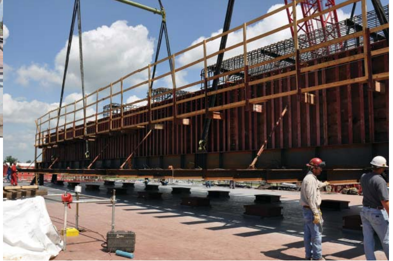
Plinth form-work being lowered onto the Vibro/Dynamics Isolators
