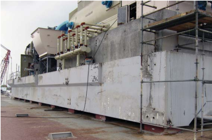
Concrete Plinth supported by the Isolators
