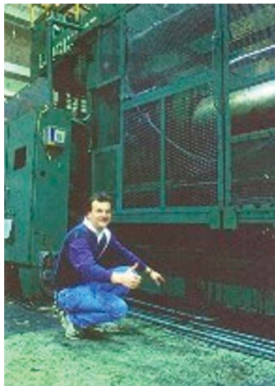
Randy Baker of Drake Molding gives the thumbs up for the installation of his 3000 ton molder installed on Vibro/Dynamics Isolators.
